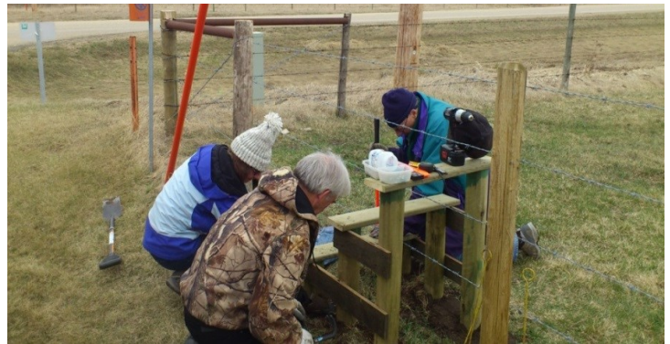
Pipestone May 2014- stile construction
