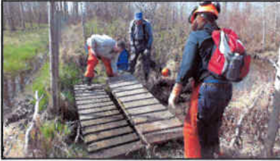
Bridge repair—Ross Creek
