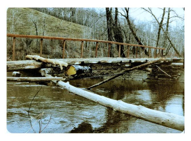
The bridge served us well for many years during which time numerous work parties raised and repaired the bridge as required. By 2017 the west bank of the river had eroded to the point where it was no longer able to support the bridge which subsequently sagged at an awkward angle at that end. We were fortunate that
