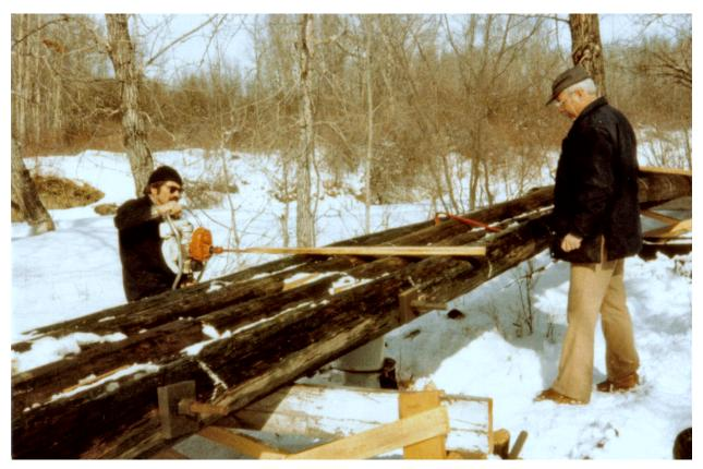
long bits for drilling through the forty inches or so of log for the steel rods, and, of course, a chainsaw was very useful, too.
